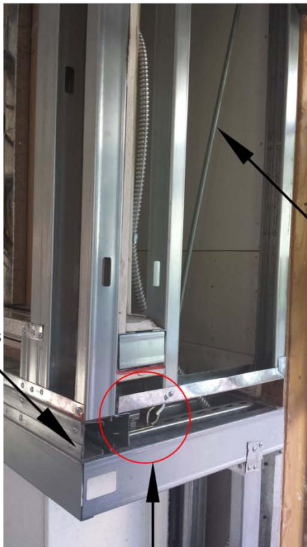
CONNECTION POINT FOR 3/4" ALL THREAD ROD TO HEADER
