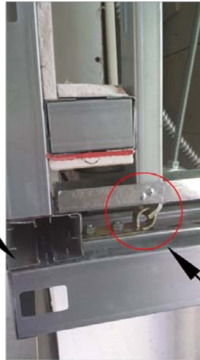
CONTINUOUS BOX HEADER SIDE VIEWS
