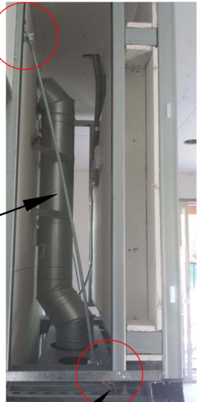
CONNECTION POINT FOR 3/4" ALL THREAD ROD TO HEADER
