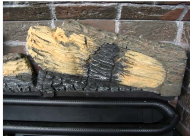
Log "B" installed correctly
