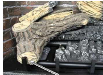
Log "G" position on front grate
